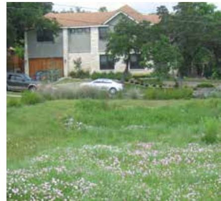
Green infrastructure, such as this drainage pond, retains rain water and reduces runoff, helping to improve groundwater quality, while reducing the need for unsightly concrete culverts and storm sewers.
