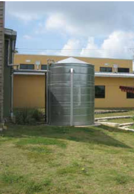
The recently constructed Twin Oaks Library in the Bouldin neighborhood incorporates many sustainable design elements including water collection, water harvesting, and solar power.
